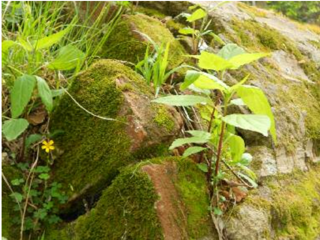
Broken column, Windsor Plantation Ruins, near Port Gibson, Mississippi Photograph by Gregory Hansen
